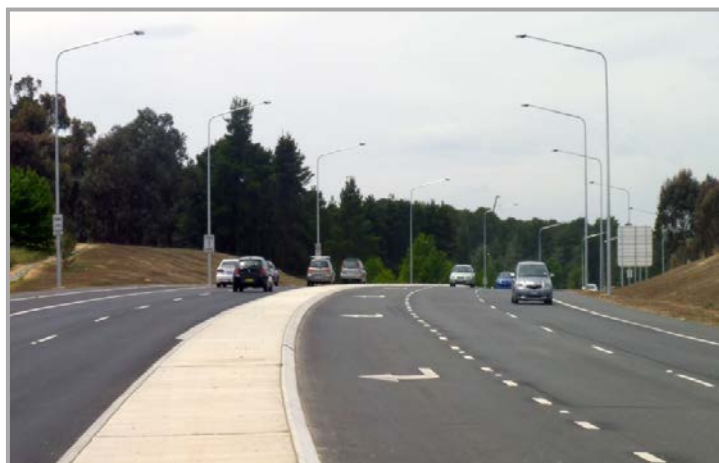
Stage 1 – Cotter Road Improvements heading towards Dunrossil Drive
