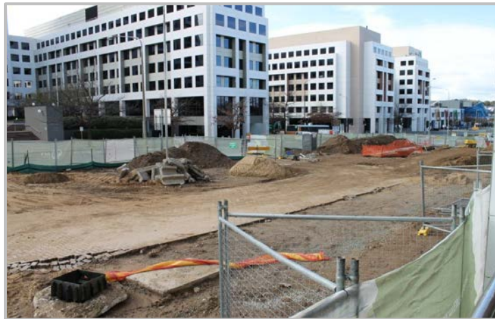
Relocation of underground cabling and services on Constitution Avenue
