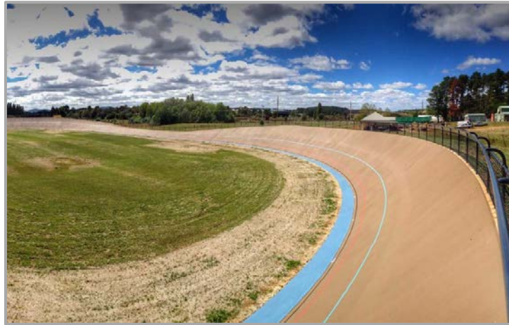
New acrylic surface as part of the Narrabundah Velodrome Upgrade
