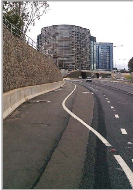
Edinburgh Avenue exit ramp and wall extension off Parkes Way
