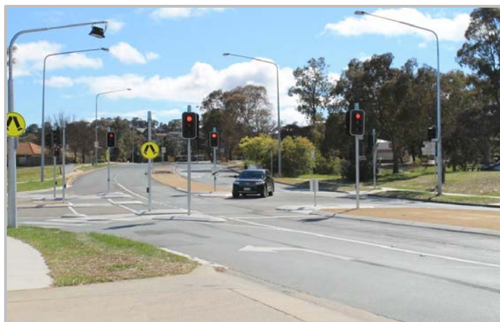
New traffic lights at Ashley Drive and McBryde Crescent intersection
