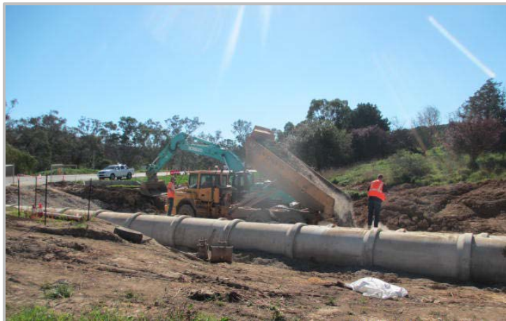
Stormwater works for Mugga Lane – Land Fill Extension – Stage 5
