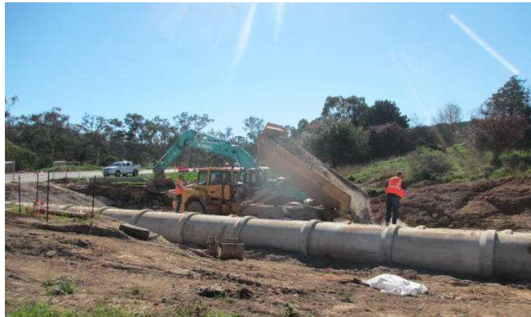
Stormwater works for Mugga Lane – Land Fill Extension – Stage 5
