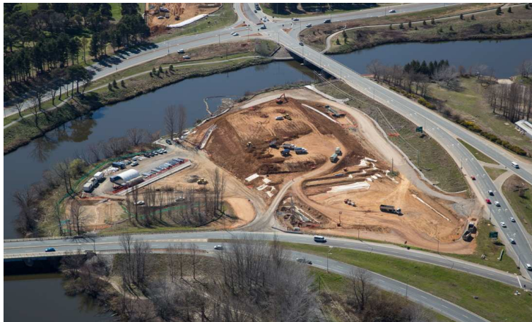
Aerial view of works underway on Majura Parkway
