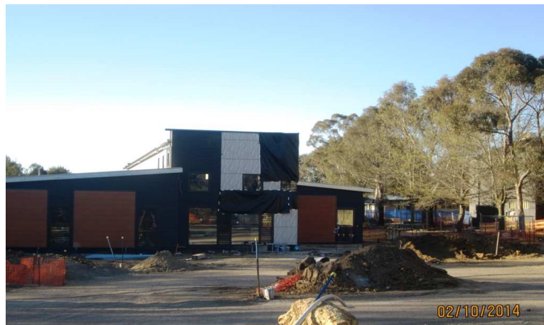
Construction of Canberra College Cares – New Building
