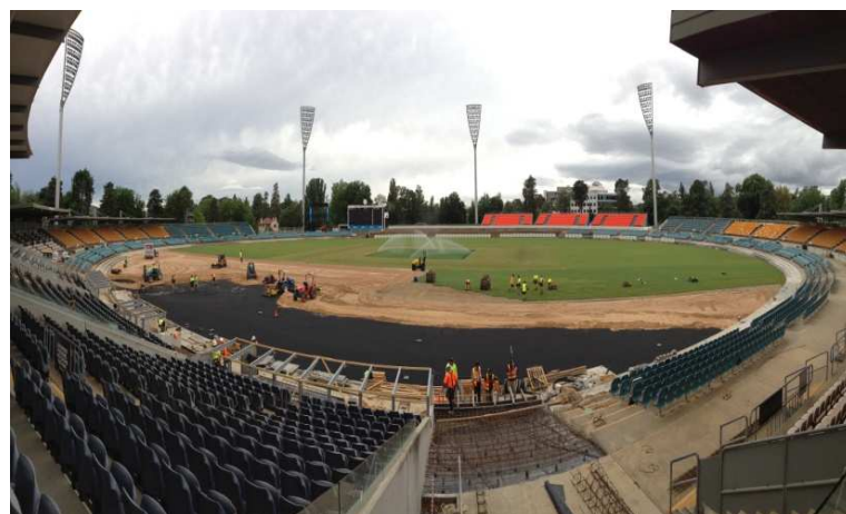
Ground works and increasing seat capacity at Manuka Oval
