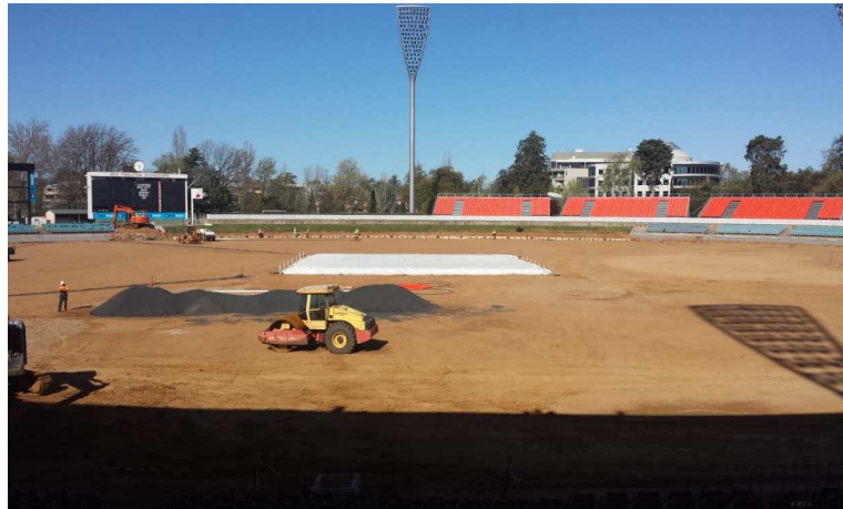
Construction works at Manuka Oval
