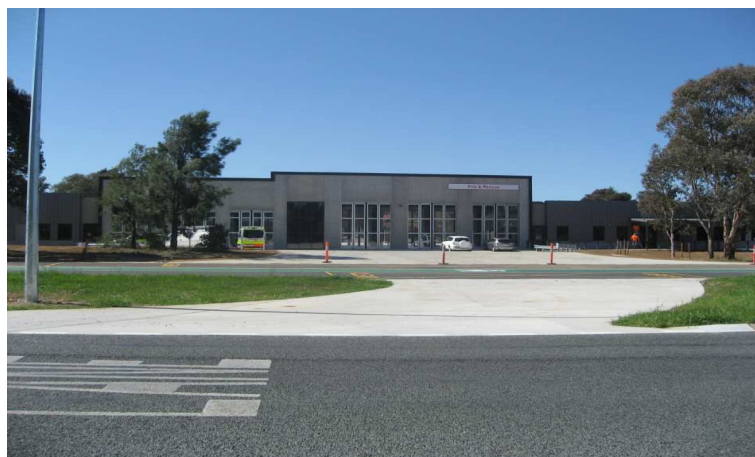
Charnwood Co-located Fire and Ambulance Station
