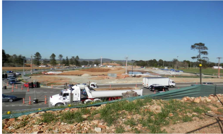
Works performed on Majura Parkway
