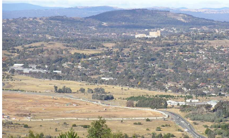
Construction of Wright as viewed from Mount Stromlo
