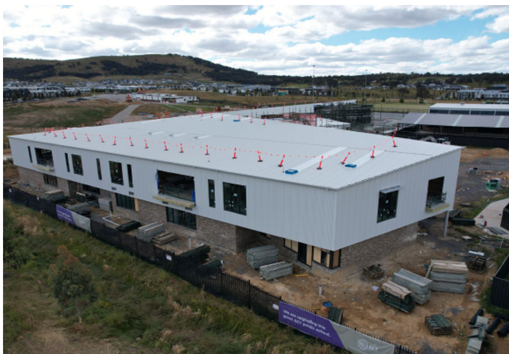
Margaret Hendry School Expansion
