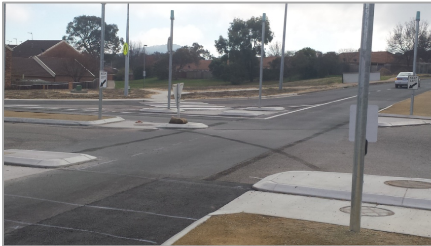
Intersection upgrade at McBryde Crescent and Ashley Drive
