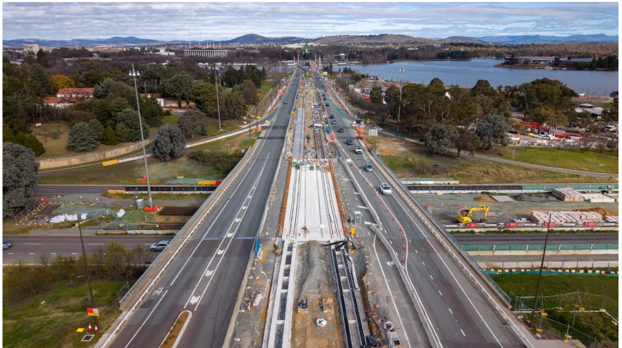
Commonwealth Avenue Light Rail Bridge over Parkes Way
