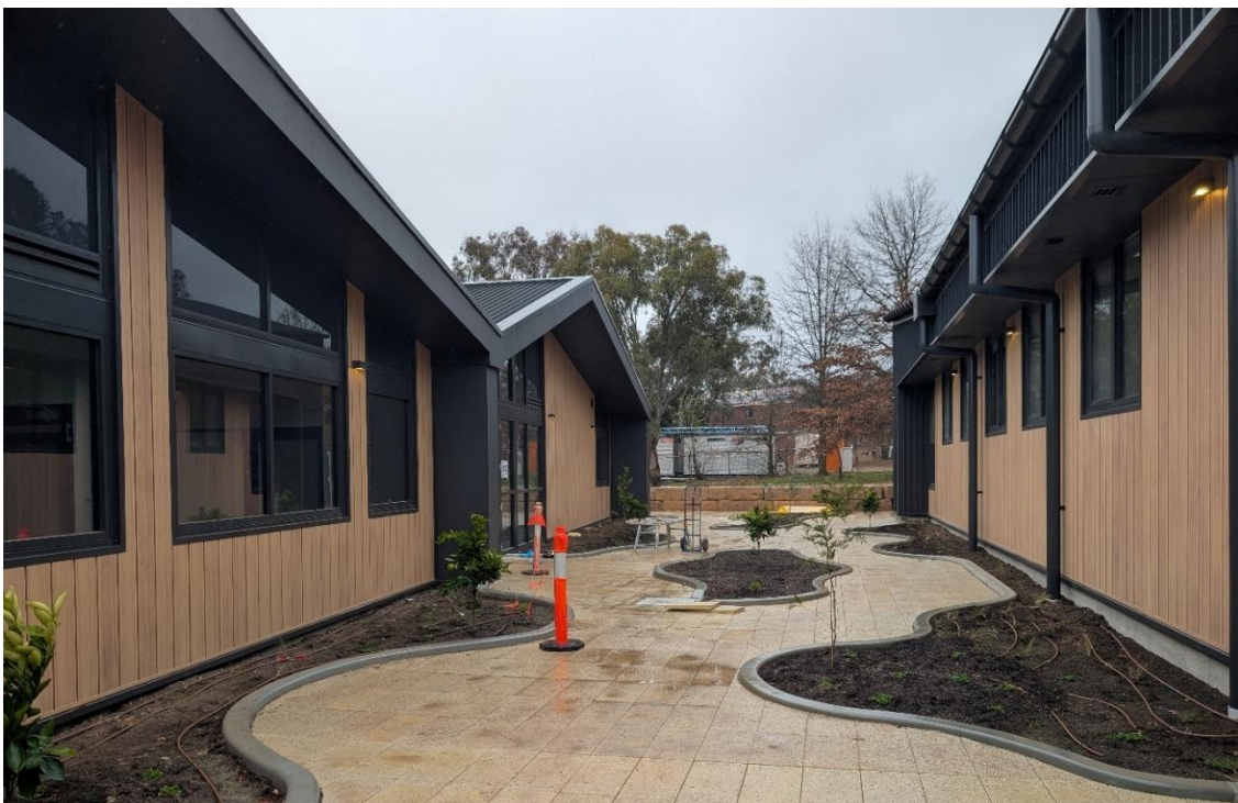
Watson Health precinct under construction
