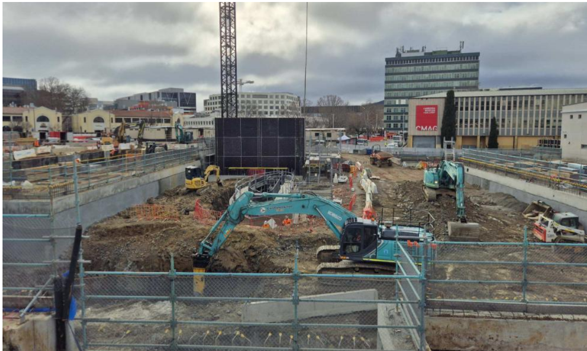
Canberra Theatre Redevelopment under construction
