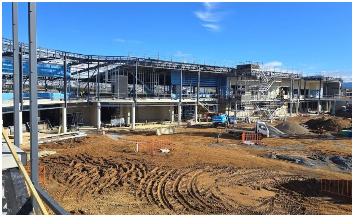
Whitlam Primary School and Early Childhood Education Centre Main Building Zone 1 under construction
