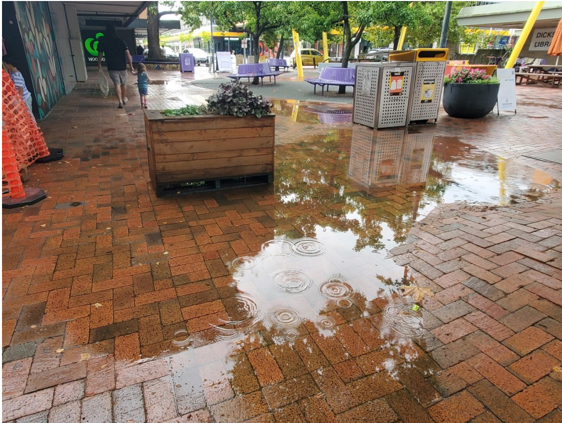
Blocked drains in Taglietti Square
