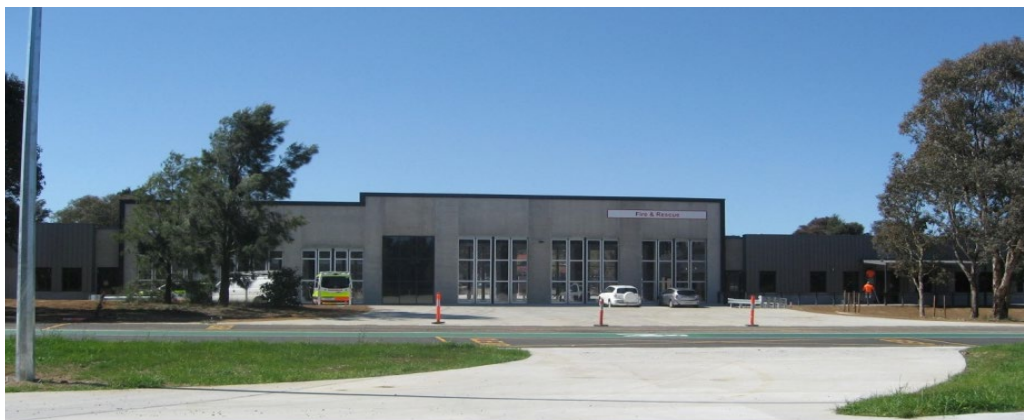
Charnwood Co-located Fire and Ambulance Station.
