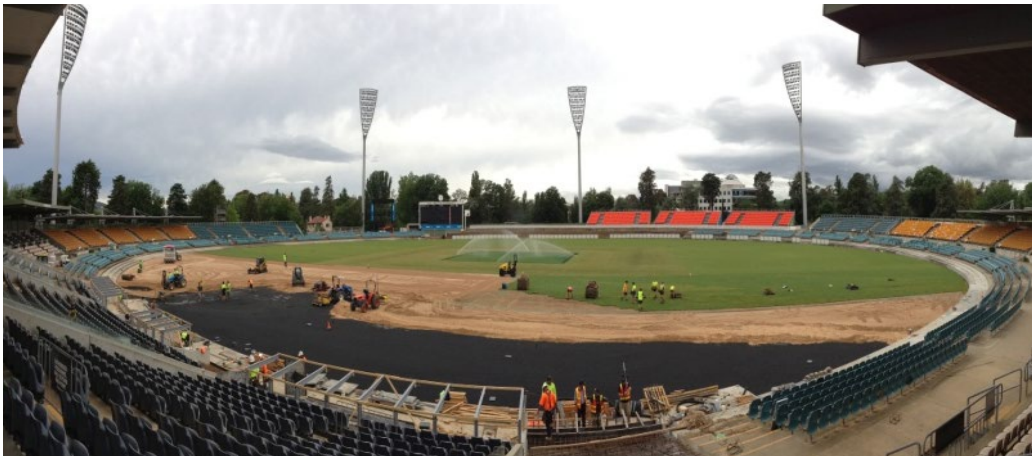
Ground works and increasing seat capacity at Manuka Oval.
