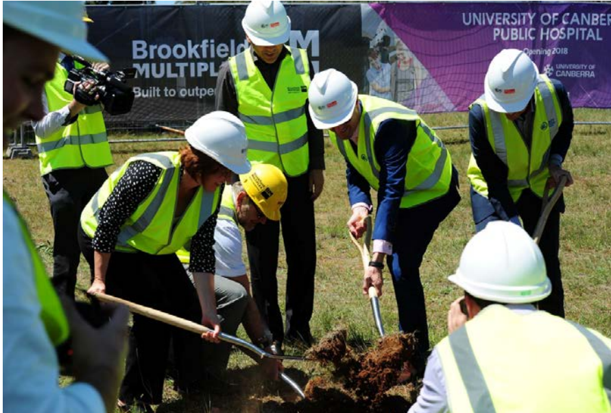
University of Canberra Public Hospital – Sod Turning
