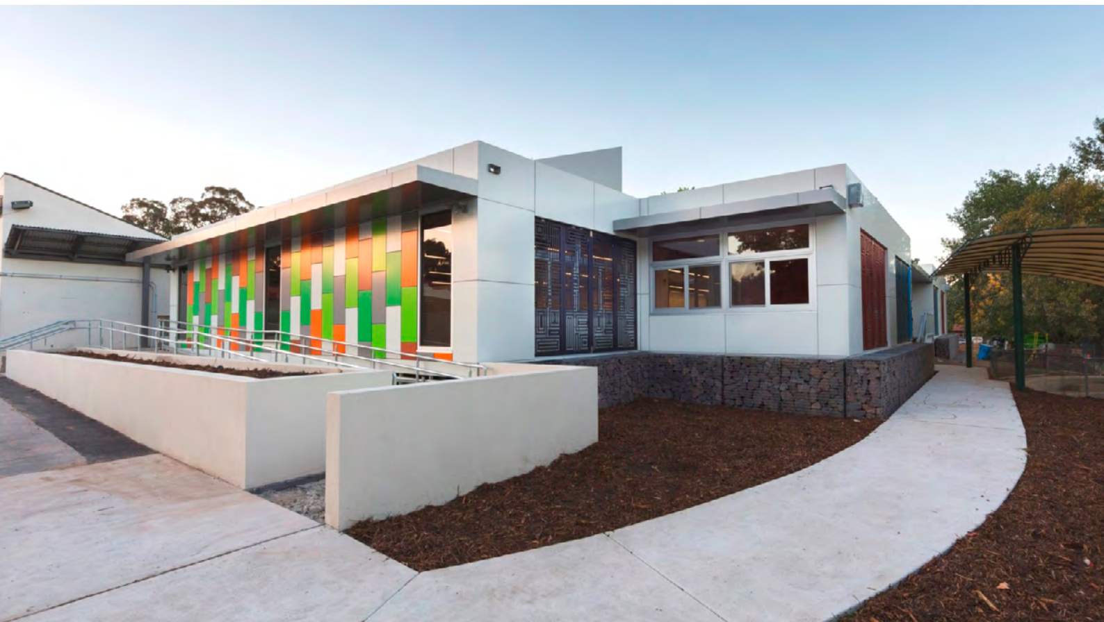
The recently completed expansion of Duffy Primary School
