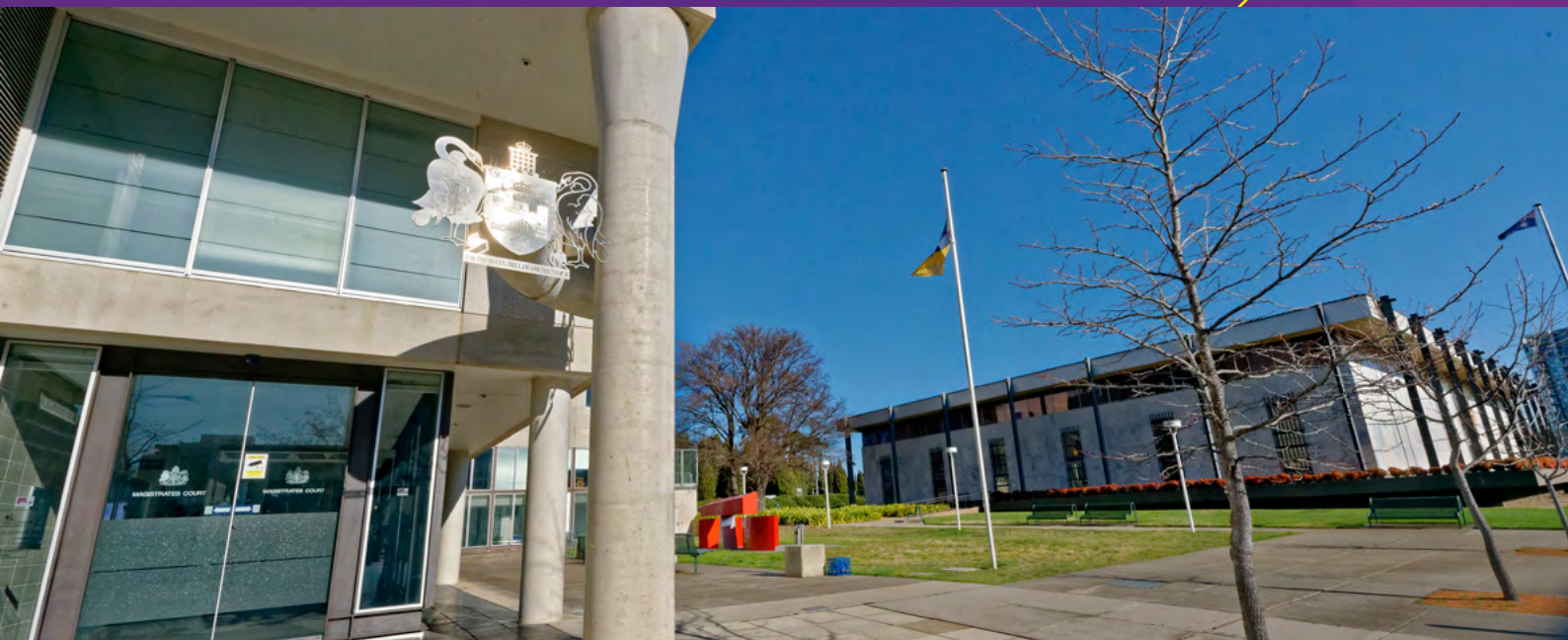
The current two distinct court buildings
