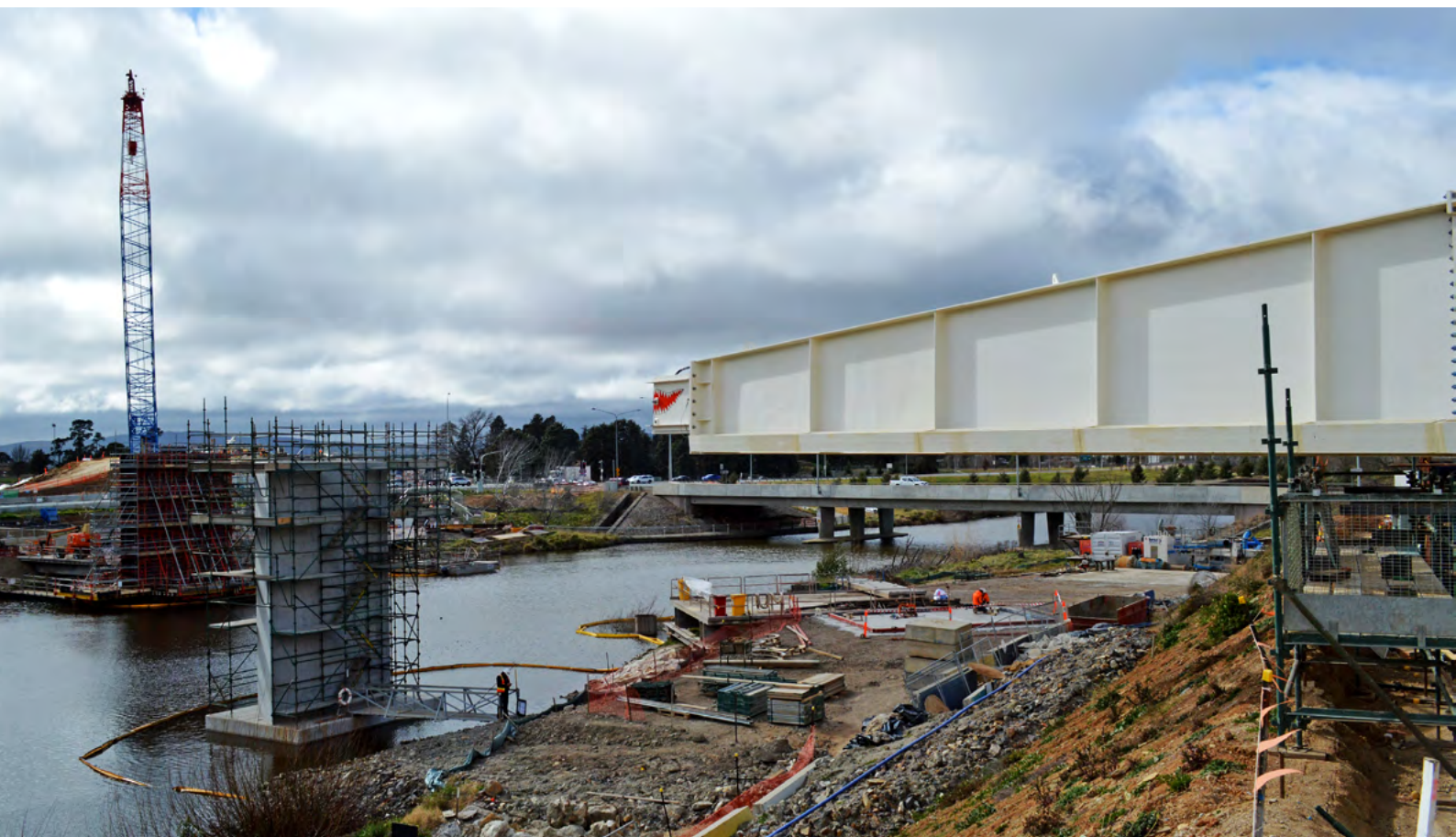
Construction of Majura Parkway's Bridge No. 1 over the Molonglo River
