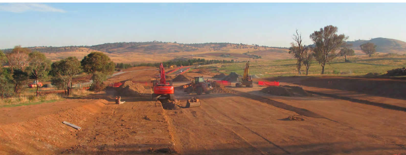
Construction in the Molonglo Valley
