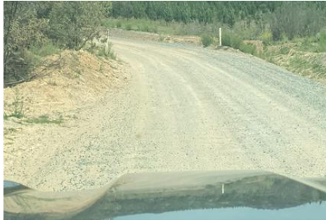
A deadly narrow, sharp & blind corner, with deep drains at the edge (>1m deep).
