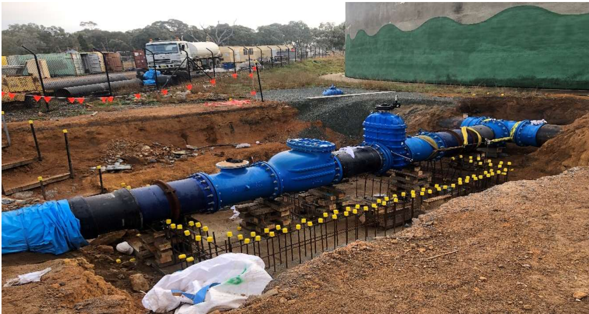
New Molonglo Valley Infrastructure – Valve pit Weetangera
