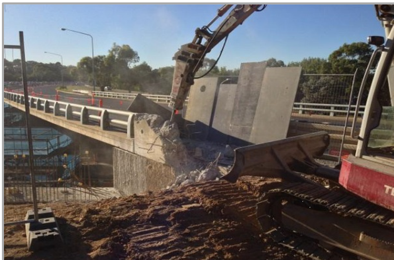
Demolition of existing guard rail on the Clunies Ross Street Bridge
