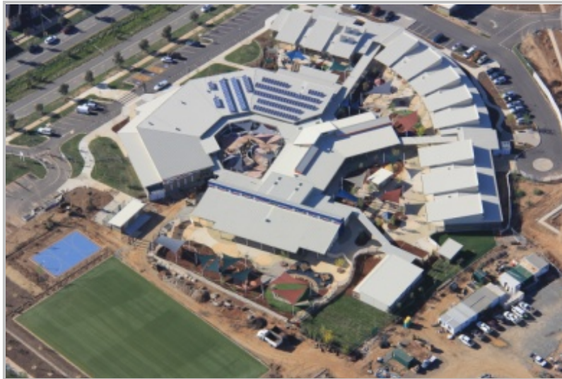
Aerial photograph of the completed Franklin Early Childhood School
