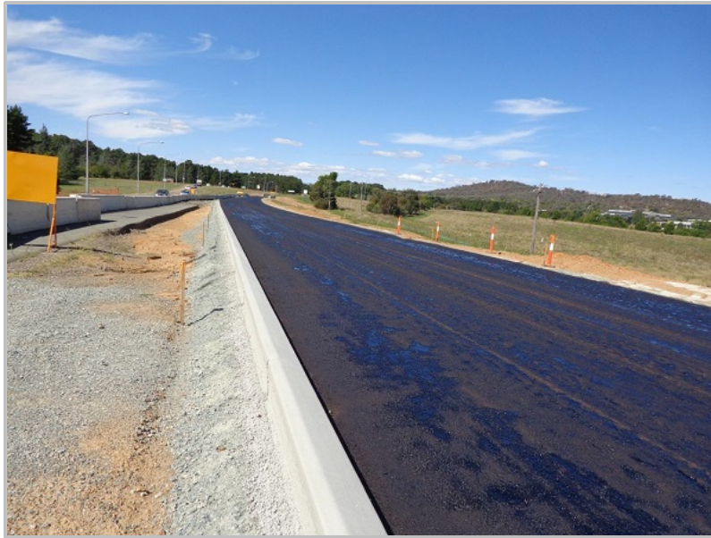
Transport for Canberra – Cotter Road Improvements asphalt laying
