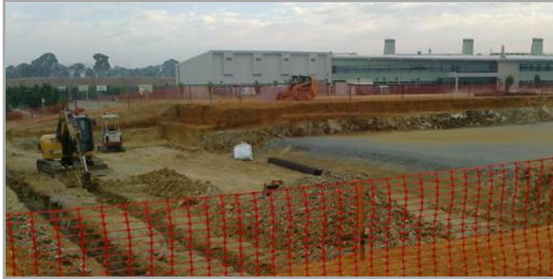
Site preparation at the Gungahlin Leisure Centre and Pool
