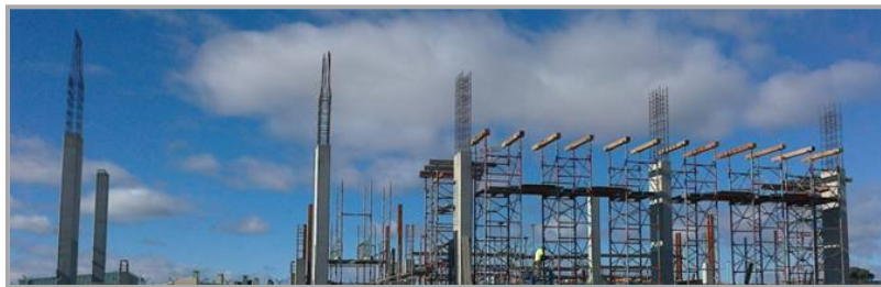
Gungahlin Enclosed Oval – Construction of Grandstand
