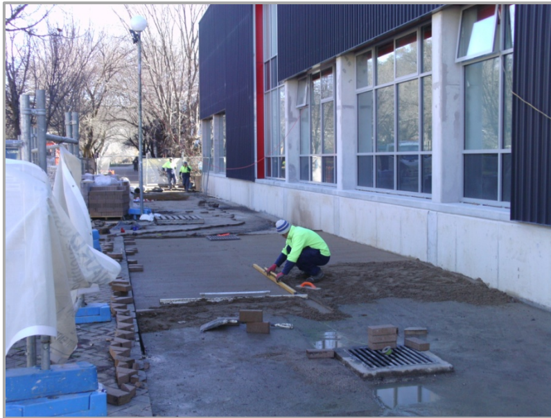
External Works at the Street Theatre Extension
