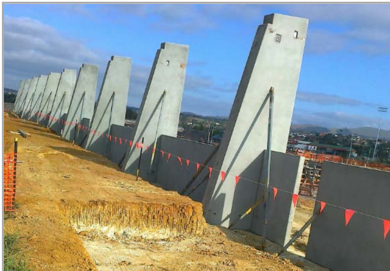
Assembled pre-fabricated panels at Gungahlin Leisure Centre and Pool
