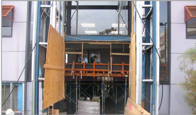
Tuggeranong Arts Centre Improvements
