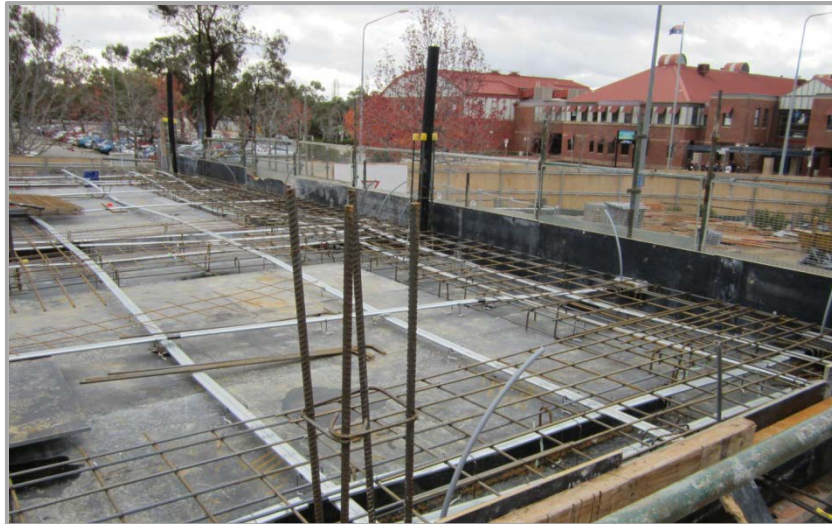
Construction of Tuggeranong Health Centre – Stage 2
