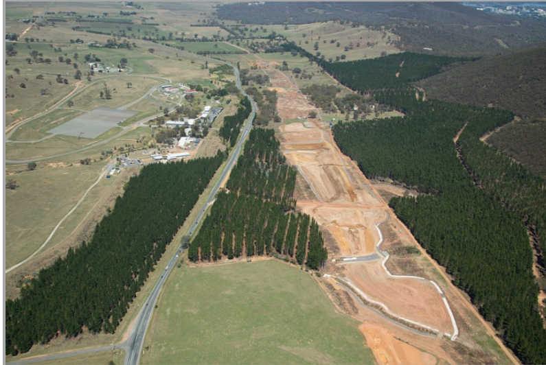
Aerial photograph of Majura Parkway construction work in Majura Pines
