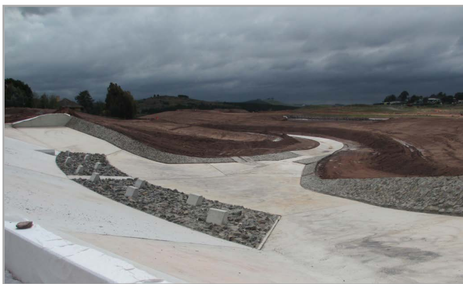
The spillway at the North Weston Pond
