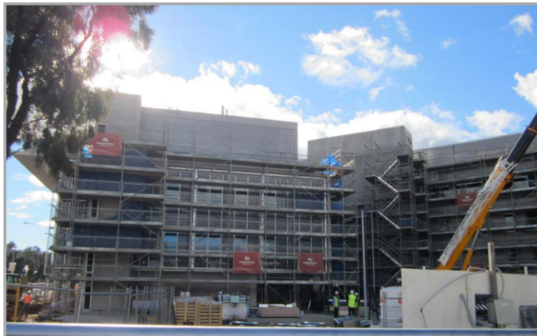
Construction of the Enhanced Community Health Centre Belconnen
