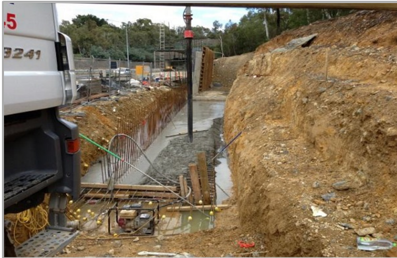
Parkes Way Widening – Pouring concrete foundations for a retaining wall
