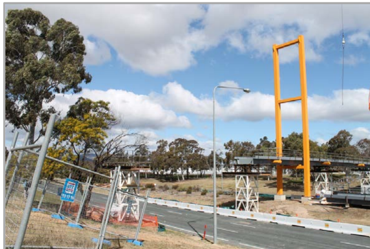
Bridge spans being installed at Namadgi P-10 School – Pedestrian Bridge
