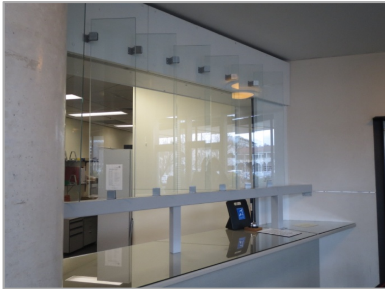
Glass Security Screens have been installed at the Magistrates Court counters
