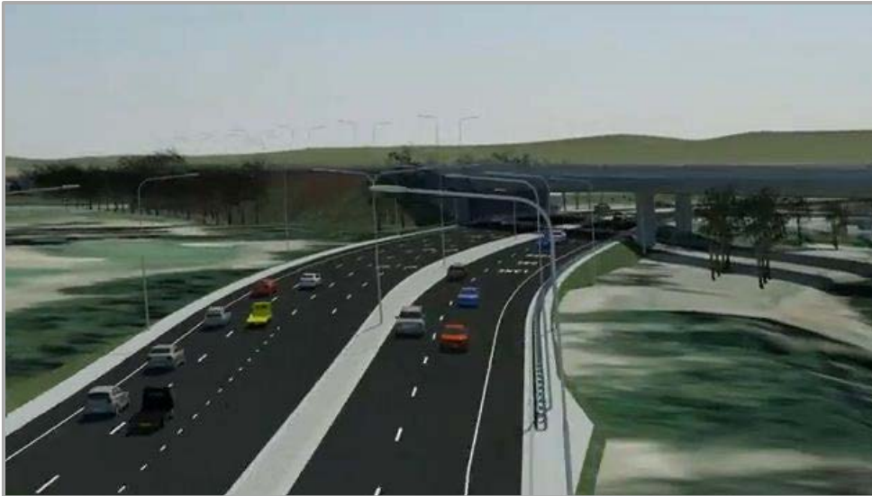
Majura Parkway – A still shot from the simulated flyover video showing the bridge that spans the Molonglo River and Morshead Drive
