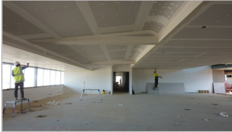
Plastering at Bonner Primary School
