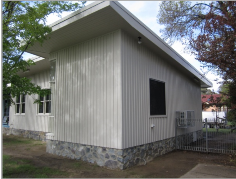
Classroom extension at Griffith Preschool
