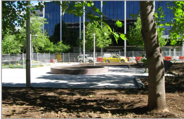
Refurbishments to the fountain and garden beds at Veterans' Park
