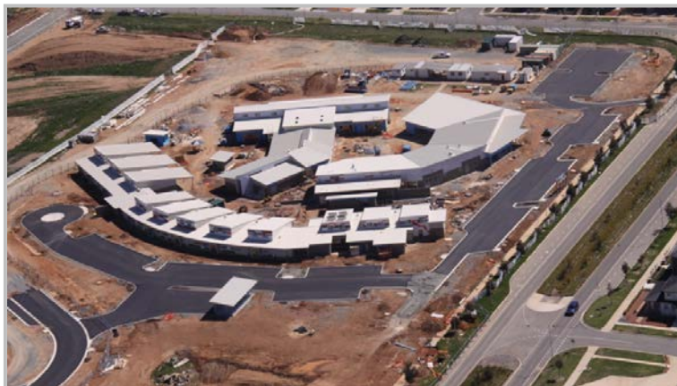
Aerial view of Franklin Early Childhood School
