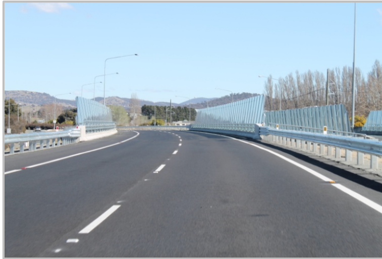
Monaro Highway Duplication – The new southbound bridge over Canberra Avenue
