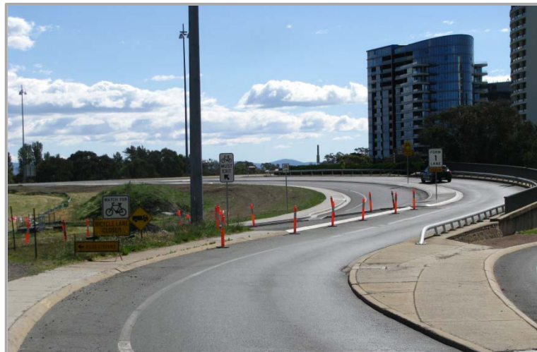
Widening of the on ramp from Parkes Way to Commonwealth Avenue
