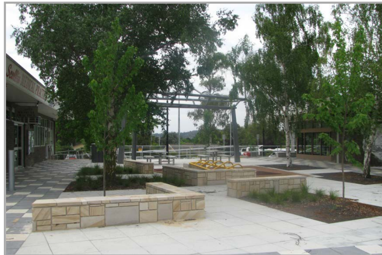
Upgrade of Scullin Shops
