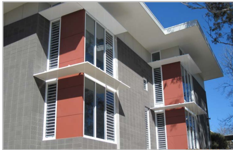
Exterior of the new classrooms at Red Hill Primary School
