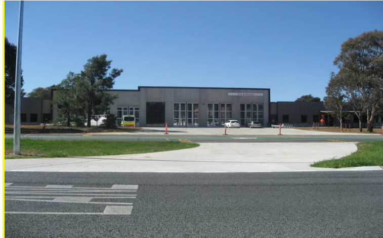
Charnwood Co-located Fire and Ambulance Station
