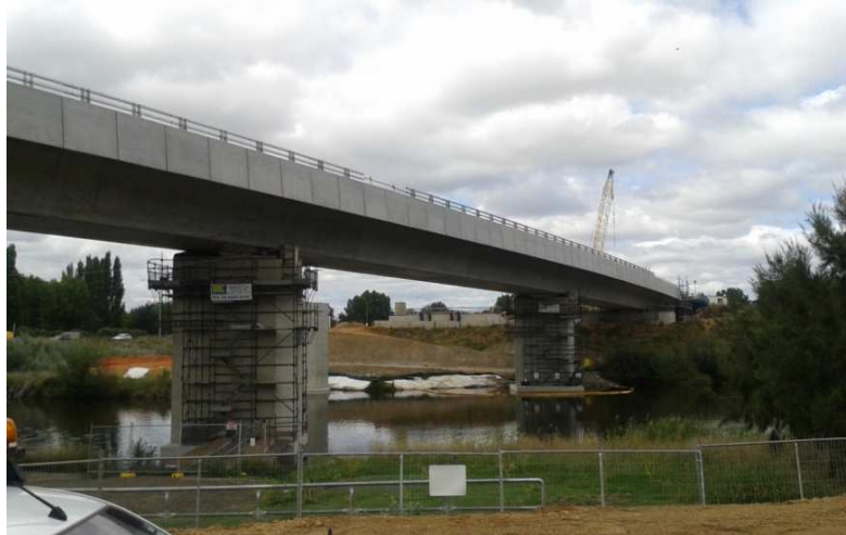
Majura Parkway Bridge across the Molonglo River
