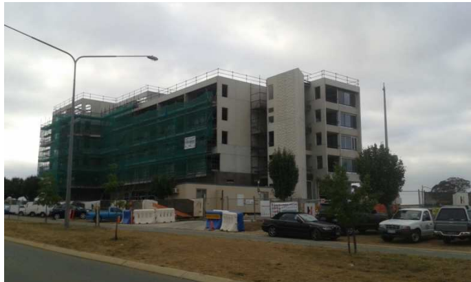
Construction of Common Ground Supportive Housing in Gungahlin
