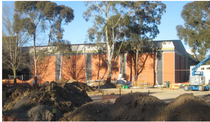
Construction of Canberra College Cares – New Building
