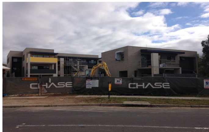
Chisholm Public Housing Units
