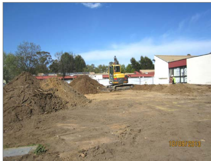
Construction site clearance at Duffy Primary School Expansion
