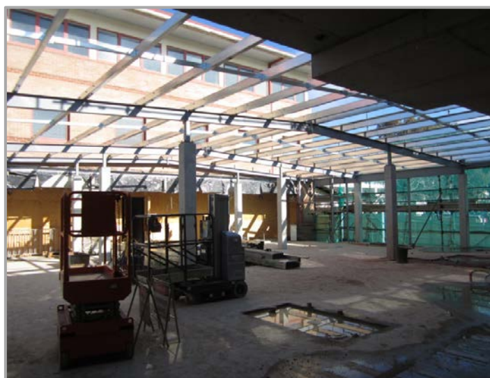
Construction of Tuggeranong Health Centre – Stage 2
