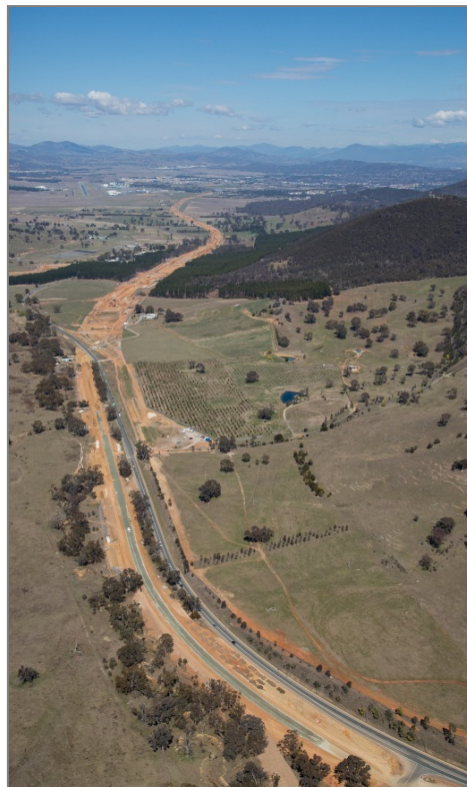
Aerial view of works underway on Majura Parkway
