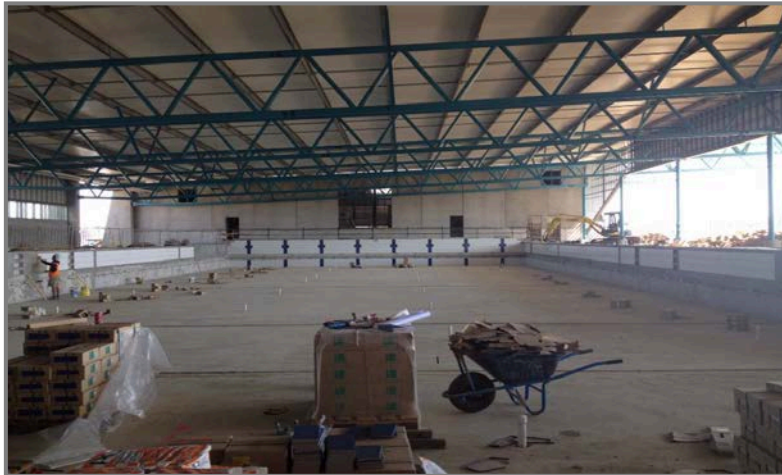
Construction of the 25 metre swimming pool at Gungahlin Pool
