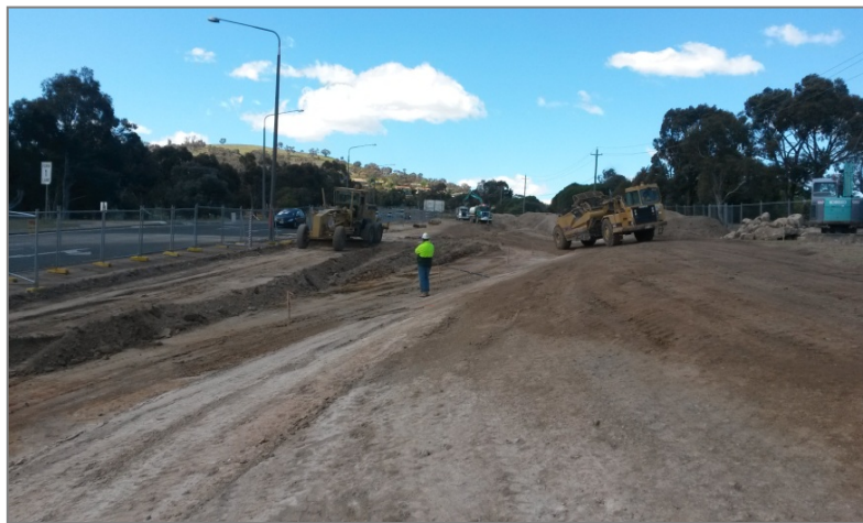
Works performed on Ashley Drive – Stage 1
