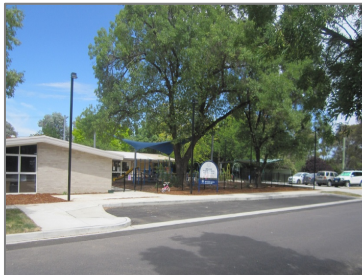
External view of Watson Preschool Classroom Extension
