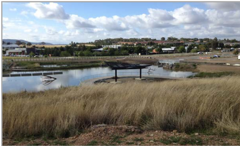
Valley Ponds and Stormwater Harvesting Scheme
