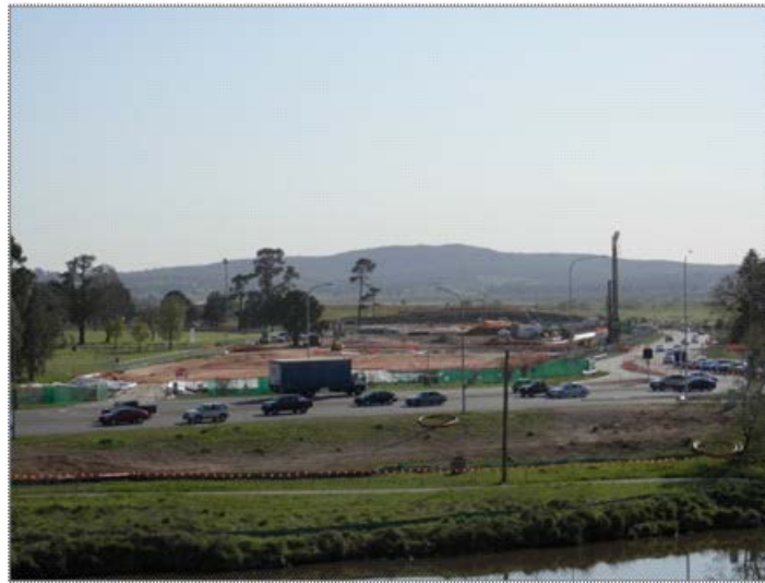
Works performed on Majura Parkway
