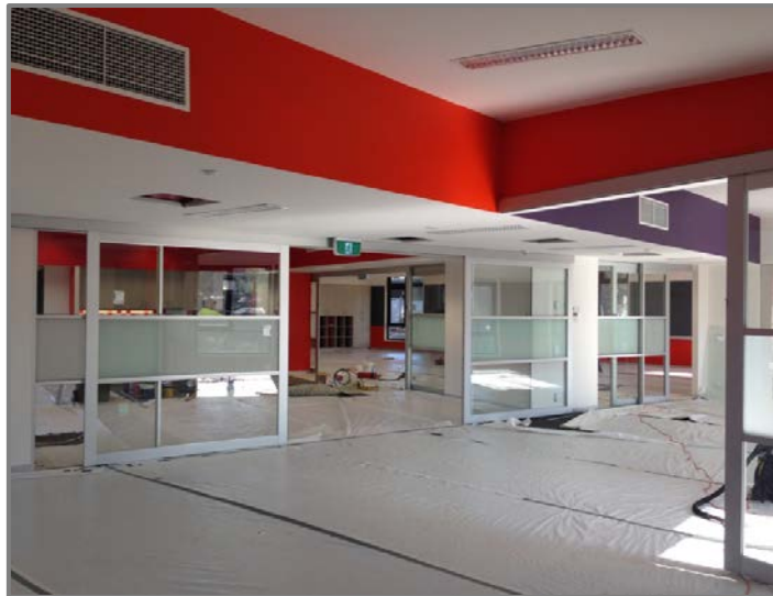
Years 5 and 6 building for Macgregor Primary School Expansion
