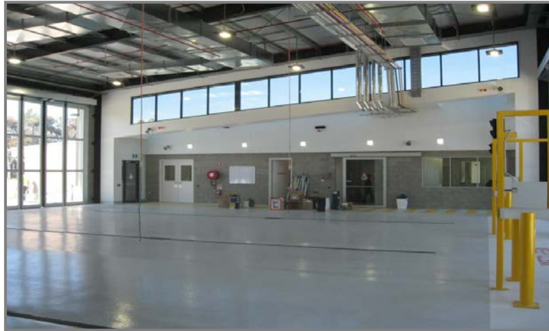
Main shed of the ESA Station Upgrade and Relocation – Charnwood Station
