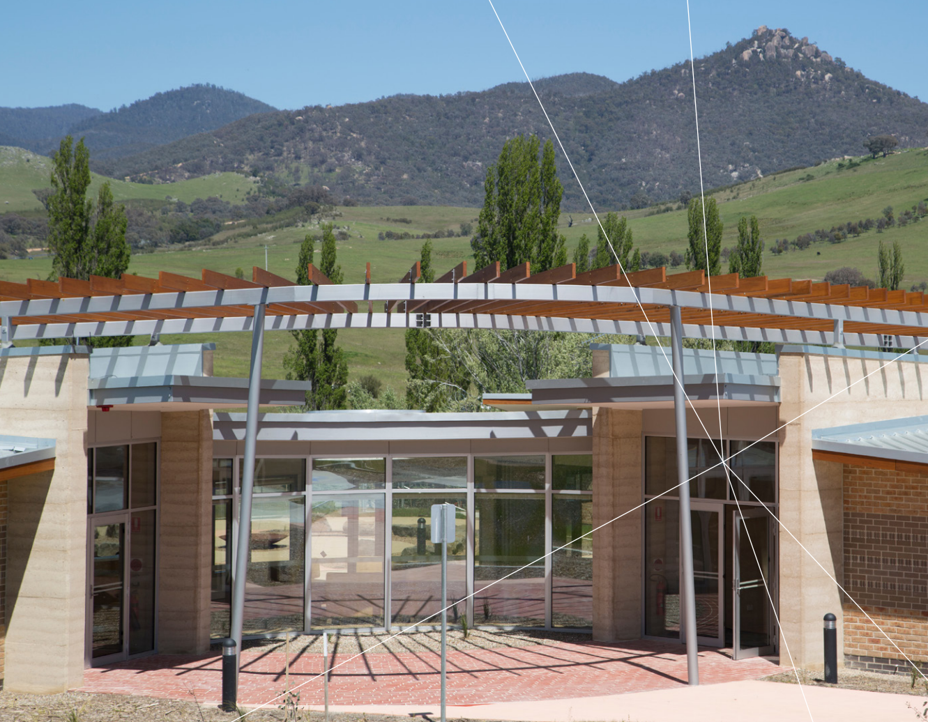
The Ngunnawal Bush Healing Farm, nearing completion, will provide a culturally appropriate alcohol and other drug residential rehabilitation service for adult Aboriginal and Torres Strait Islander people in the ACT
