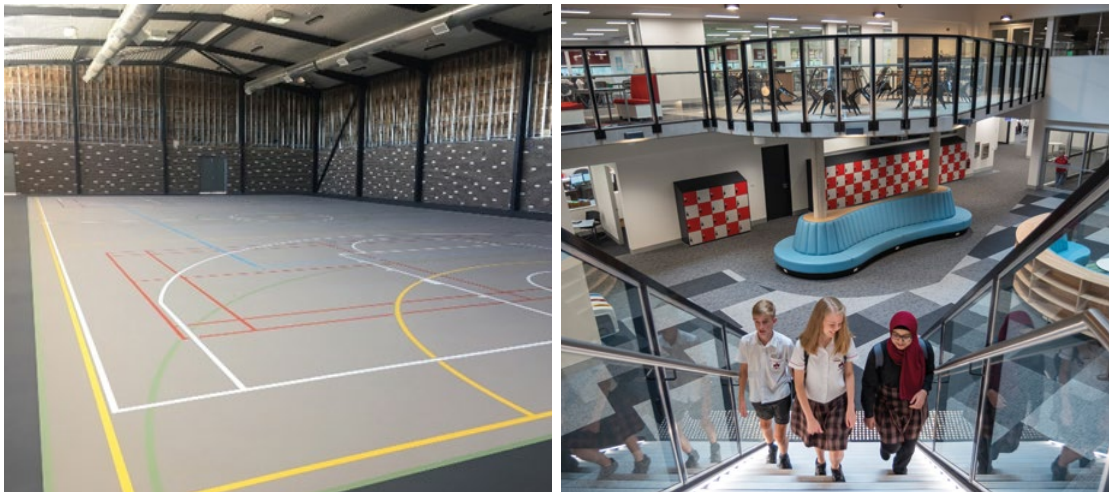
Margaret Hendry School gymnasium (left) and Belconnen High School contemporary learning spaces nearing completion (right)
