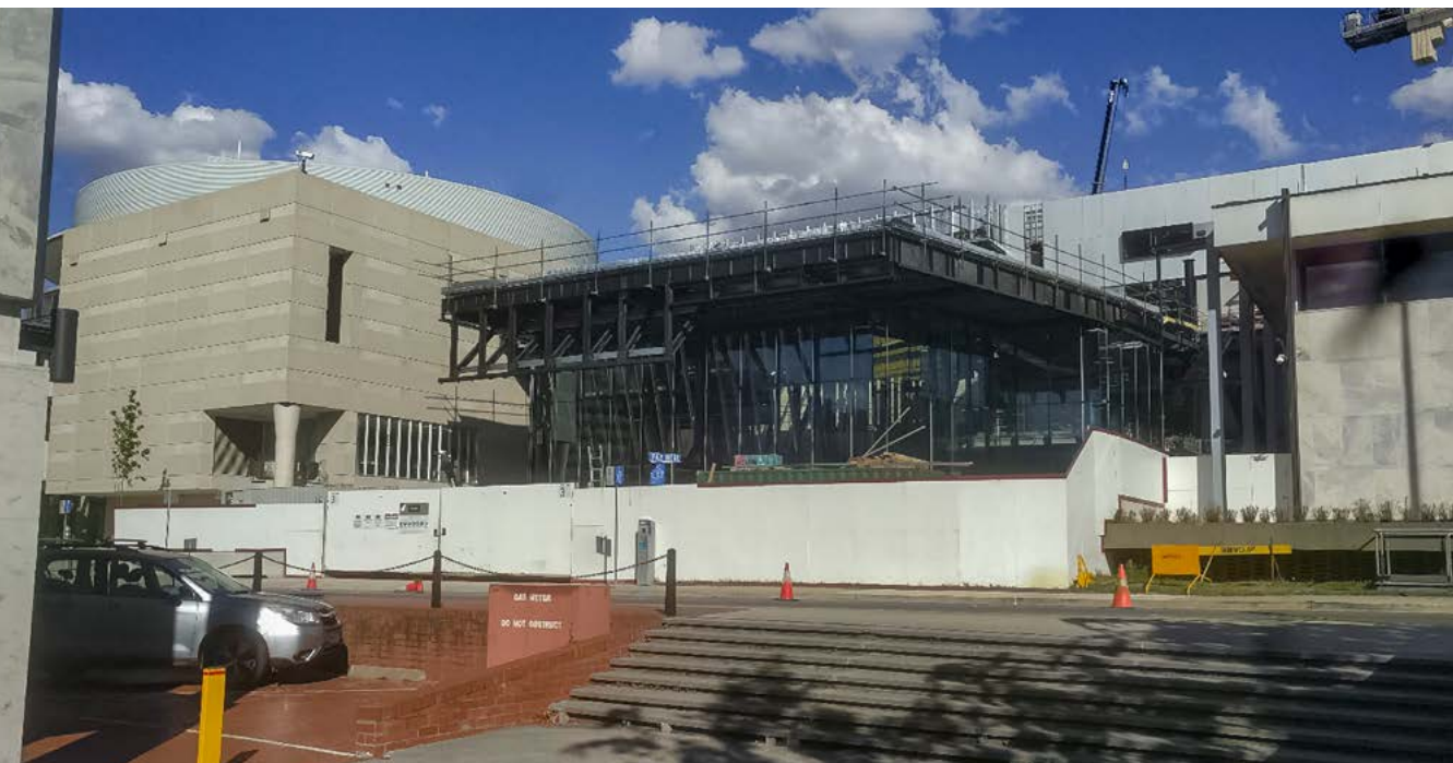
Construction of the new ACT Law Courts facilities
