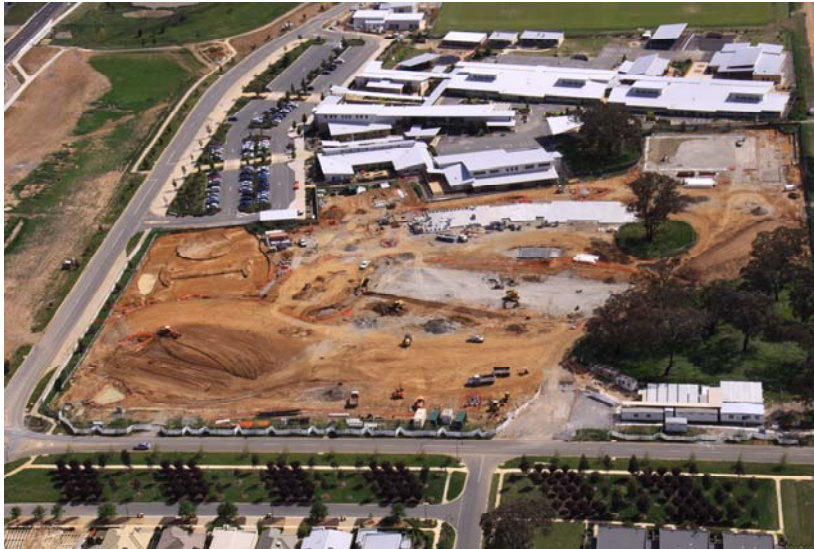
Site establishment and slab works underway at Harrison High School
