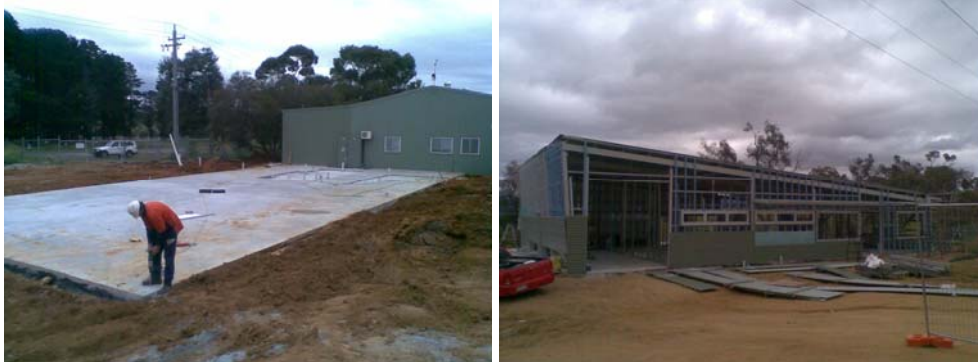
Works progressing on the Jerrabomberra (left) and Rivers (right) Sheds
