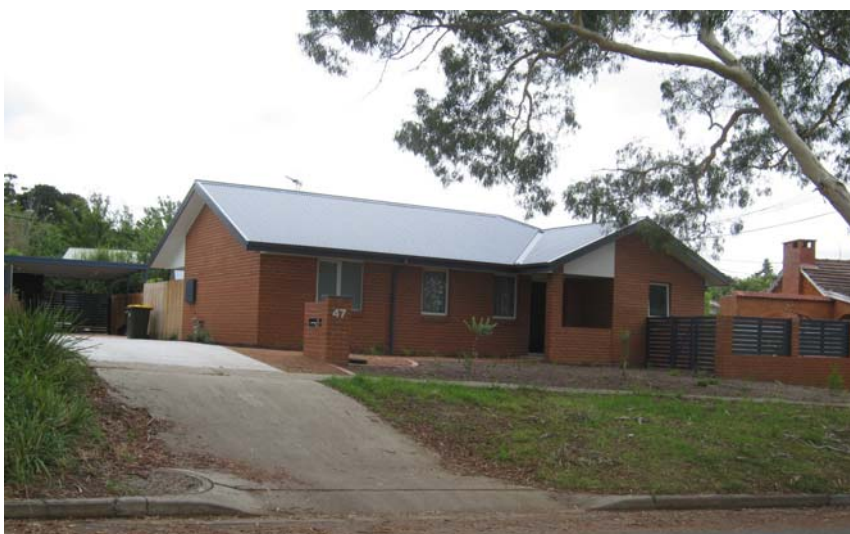
Completed social housing dwellings in O'Connor ( Nation Building and Jobs Plan )
