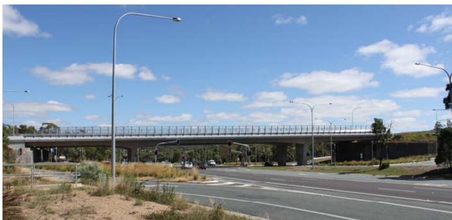
The Belconnen Way Overpass section of the GDE
