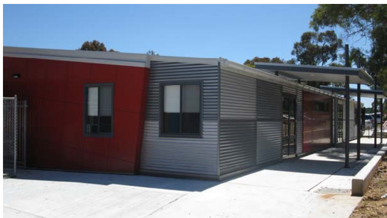
Fraser Primary School's new multi purpose building
