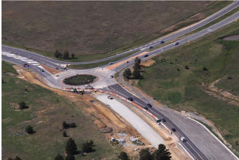
Looking south during construction of the westbound carriageway of Lanyon Drive
