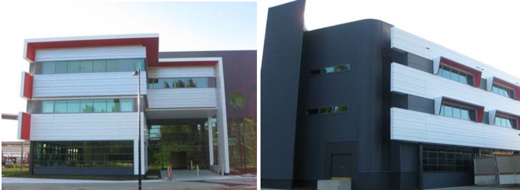
External view of the Electrotechnology Building at CIT Fyshwick
