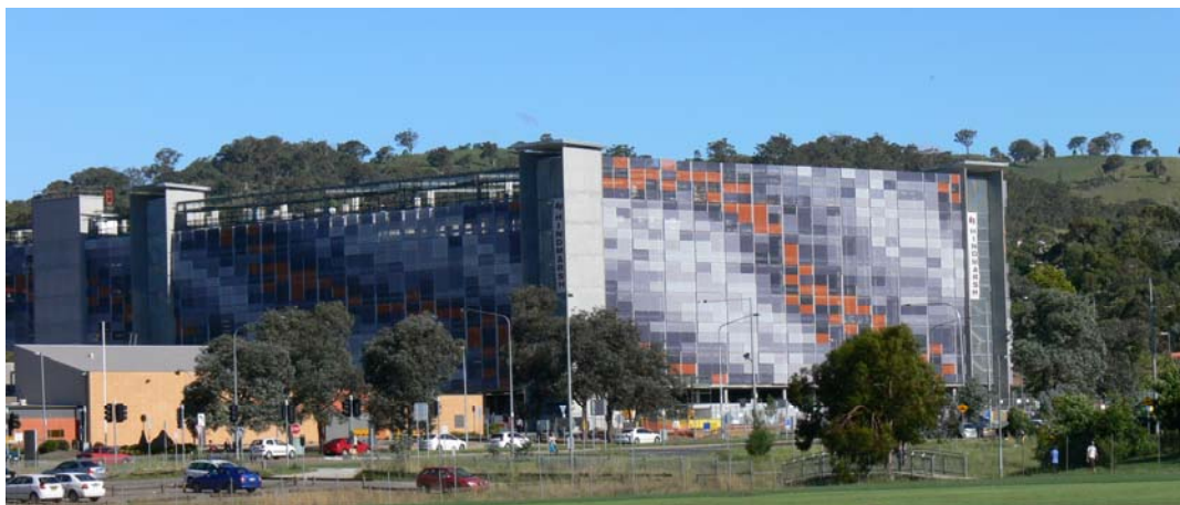
The exterior of the multi-storey car park at the Canberra Hospital
