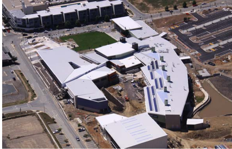
The near fully completed Gungahlin College site
