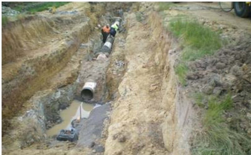
Progressing works on the Bonner sewer
