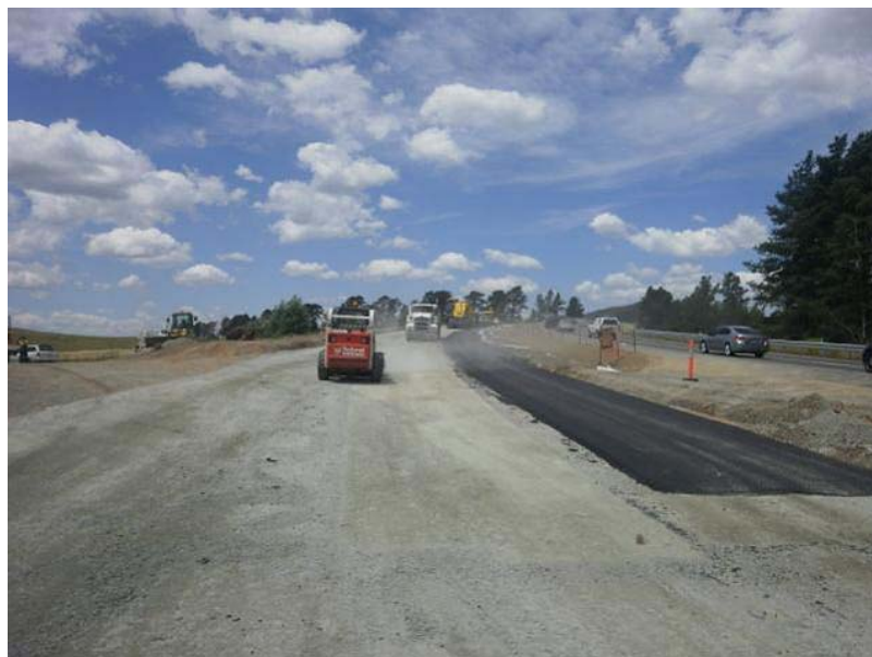
The laying of new asphalt pavement on Lanyon Drive
