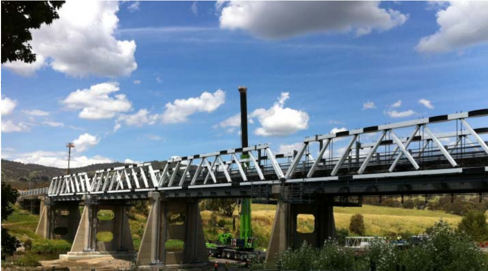
The completed installation of new trusses on the Tharwa Bridge
