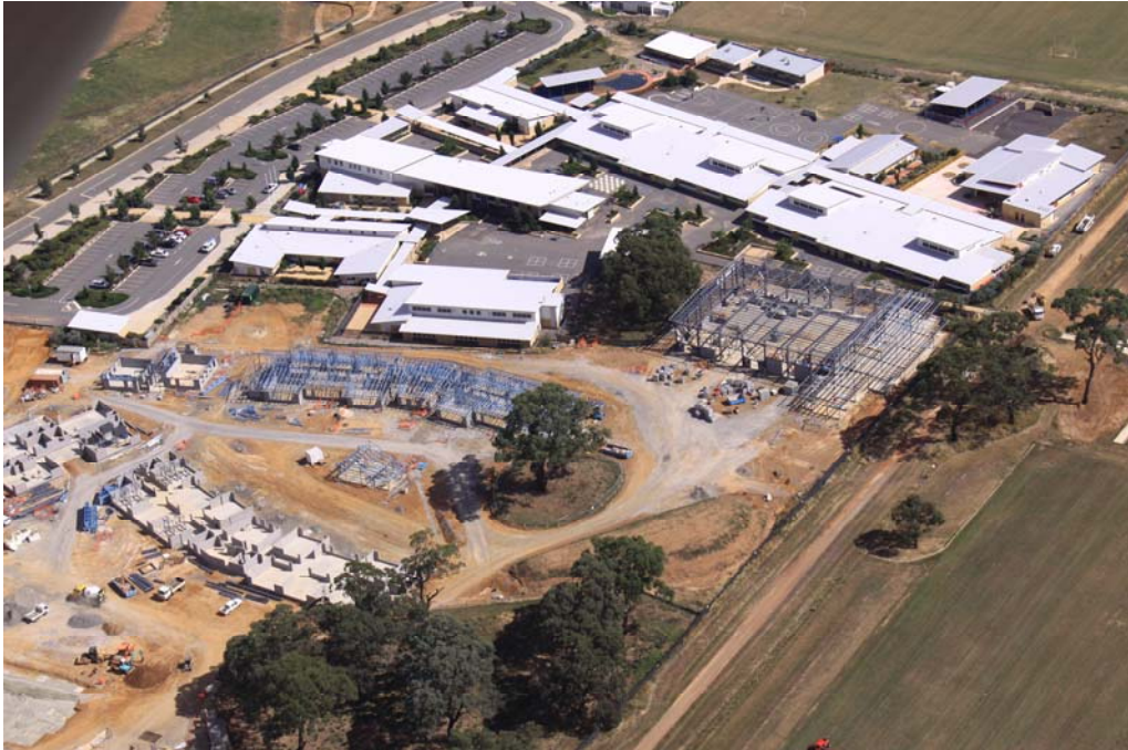
Construction progressing on first stage buildings at Harrison High School
